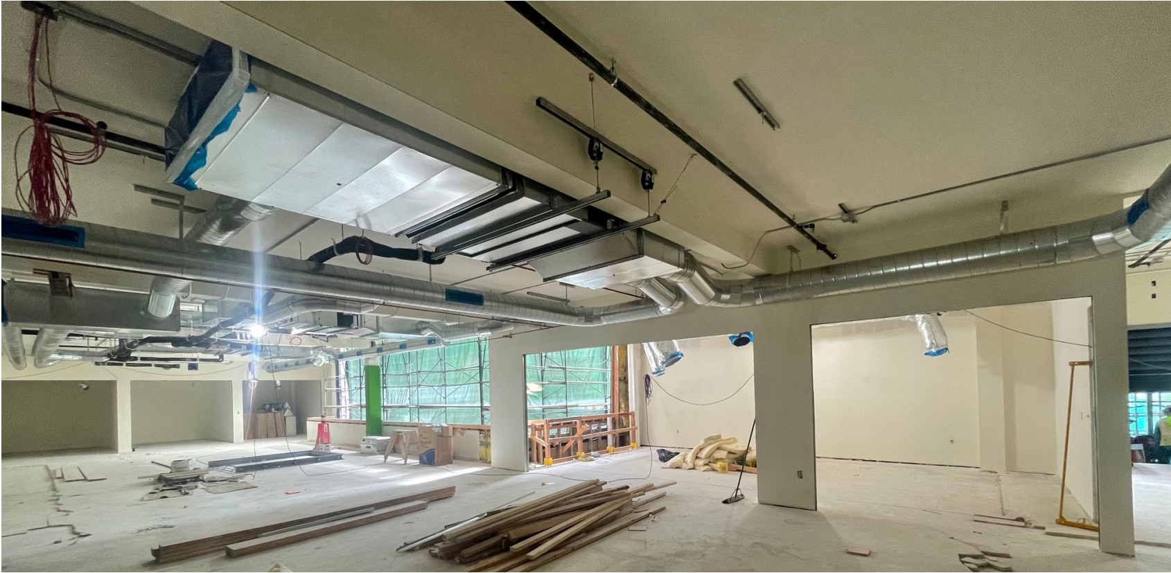
10240 Sorrento Valley Road | Construction Currently Underway
